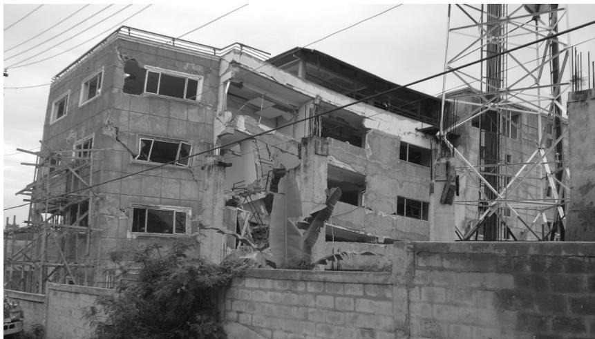
Figure 4. Damage to recently built commercial building approximately 0.5 kilometer west of HVCV. The building was later demolished.
