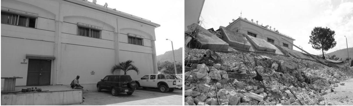
Figure 3a. (left) Canape Vert Voila cell phone facility; 3b. (right) collapse of retaining wall in parking lot. The face of the building seen in the photograph is aligned roughly N-S; the battery racks discussed in this study are located on the ground floor, in a large room behind the doors seen at left in Figure 3a.
