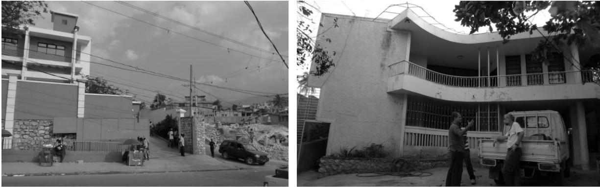
Figure 2a (left) A good-quality commercial structure in which MMI V-VI is estimated based on an eyewitness interview; 2b (right) a private home, masonry C construction, for which MMI VI is estimated. The structures on both sides of the structure shown in 2a collapsed catastrophically, as did a school building adjacent to the house shown in 2b.
