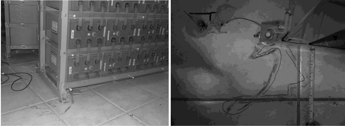
Figure 5a. (left) Rack of batteries that was moved across the floor during the mainshock. The near (short) edge of the front rack is aligned roughly N-S, with the closest edge towards the south; 5b (right) close-up of scratches left on tile, including pen marks drawn to indicate inferred trajectory. (The loop is inferred to have been left by a remnant of the bolt that was dragged as the rack moved)
