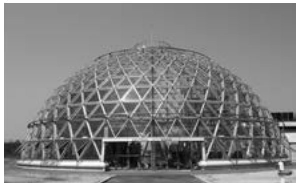
Arid Land Dome was constructed in 1998 to enhance the efficiency of research at ALRC.
