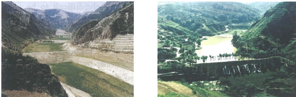
Fig. 6.1 Check dam (earth-fill dam) in Loess Plateau for mitigating the soil erosion and the sediment transportation
