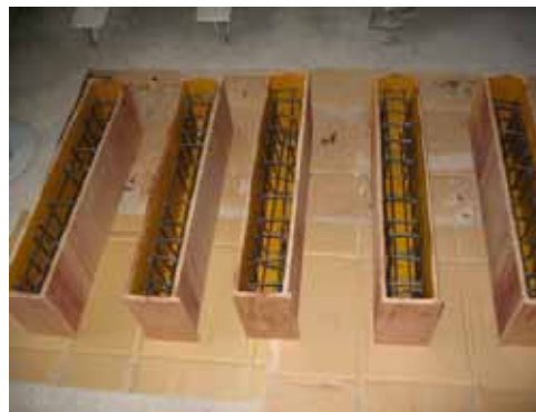
Photo 3.8: Moulds containing the reinforcement of concrete beams
