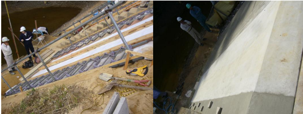
Fig 2.10 Earth dam repair with ECC in Tottori
