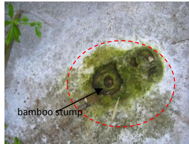
Fig.3.2.10. Circular hole on mortar plate
