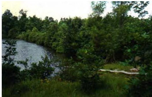
Fig.2.1. Dam with inspection-hindering trees in Tennessee[6]
