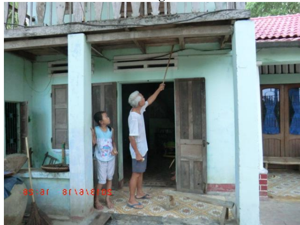
Experienced highest flood depth level of Ngo Van Quang's house, Tay An village
