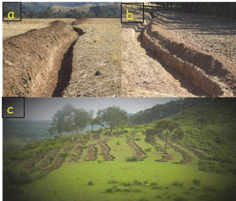
Figure 4- 5 Commonly implemented soil and water conservation measures for major land uses in the humid highlands of Ethiopia: (a) fanyajuu, (b) a soil bund on cultivated land (c) and trenches on a hillside of bush and grassland.
