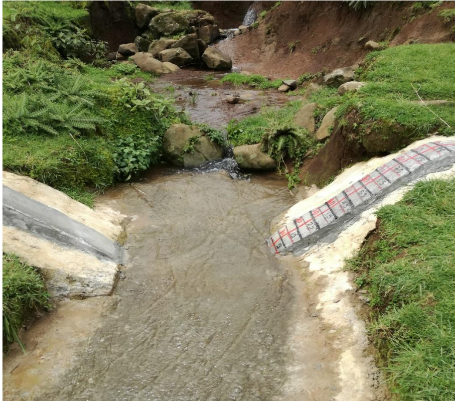
Figure 4. 5 Weir structure to monitor sediment yield from gully cross-section.
