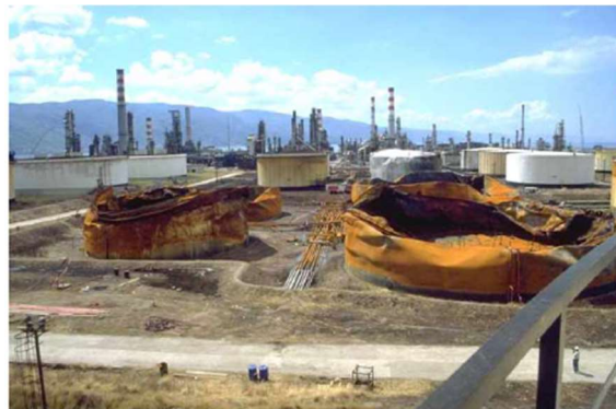
Figure 1.9 Tanks Collapsed due to Fire Accident (1999 Kocaeli Earthquake) [12]
