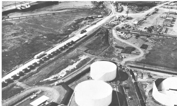
Figure 1.4 Damage to Structures in Port Area, Including Petroleum Tank (Lower Right) by Vibration and Ground Fractures (1964 Great Alaska Earthquake) [5]
