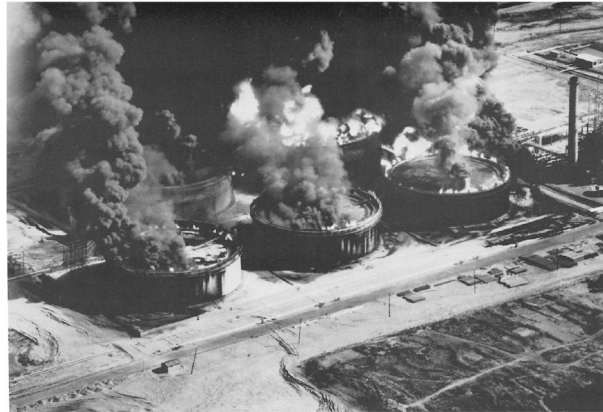
Figure 1.6 Fire Accident of Oil Storage Tanks due to Sloshing (1964 Niigata Earthquake) [8]
