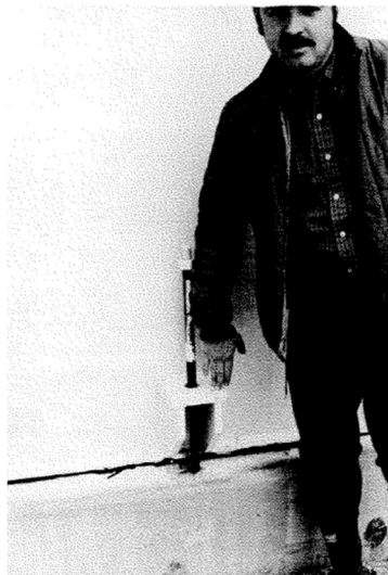
Figure 1.13 Anchor Bolt of 6,600 kL Water Tank (Anchor bolt was pulled up 35.5 cm.) [19]
