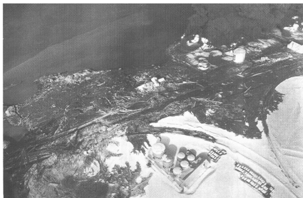
Figure 1.5 Fire Accident of Fuel Storage Tanks (1964 Great Alaska Earthquake) [6]
