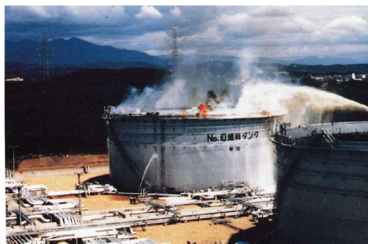
Figure 1.7 Fire Accident of 35,000 kL Oil Storage Tank (1983 Nihonkai-Chubu Earthquake) [9]
